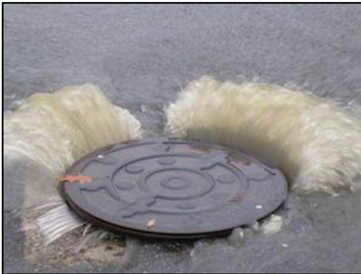
Examples of sanitary sewer overflows. Pictures courtesy of City of Raleigh, North Carolina.
